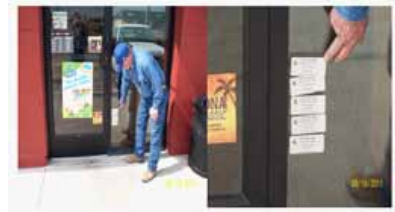
Building Inspectors check placement of signs and stickers
