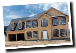
APA's Simplified Bracing Method permits designers to take advantage of the strength found in shorter wall sheathing segments and count them as bracing segments.
